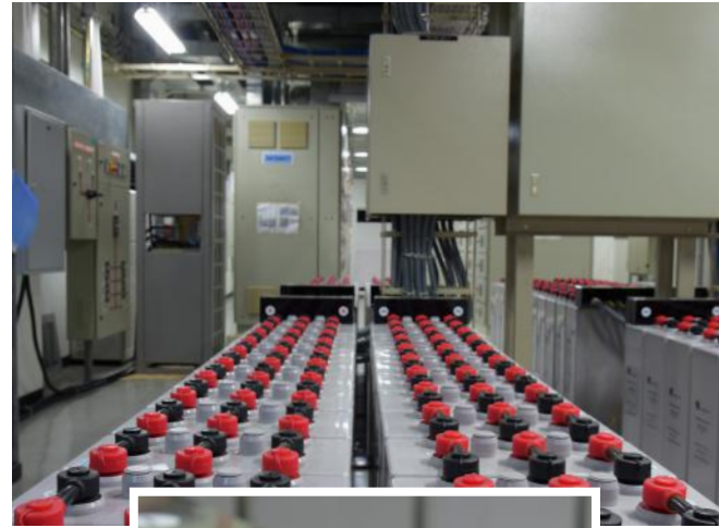
Battery Storage for Cellular Communications Switchboard
