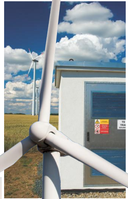
Wind Power Transformer Station
