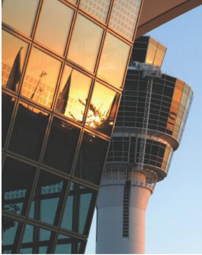
Air Traffic Control Tower
