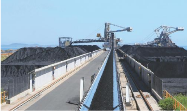
Dock side Coal Conveyor
