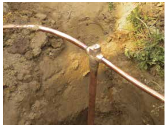
GT Cadweld connection
