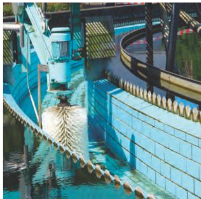
Sewage Water Treatment
