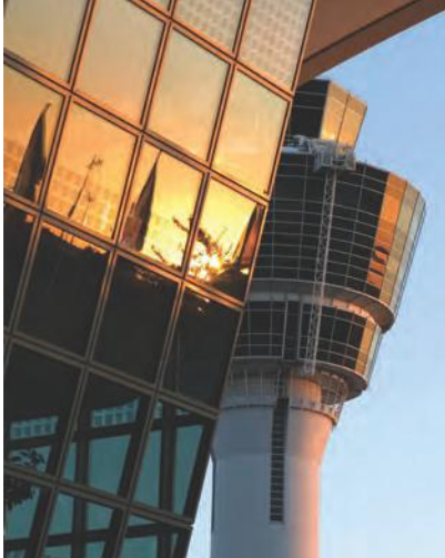
Air Traffic Control Tower
