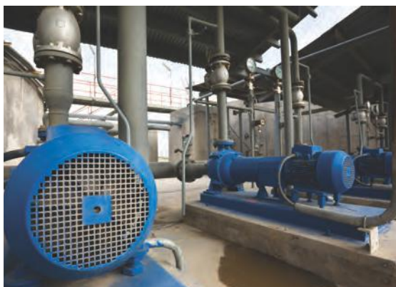
Water Pumping Station
