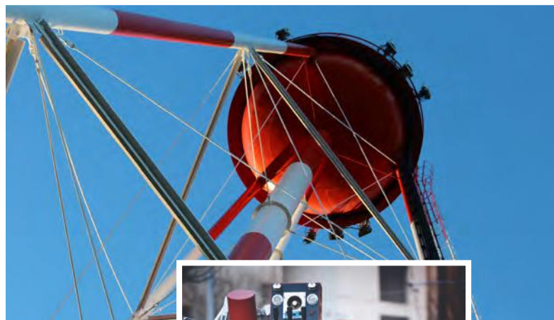
Water Tower with Cellular Radios and Antennas
