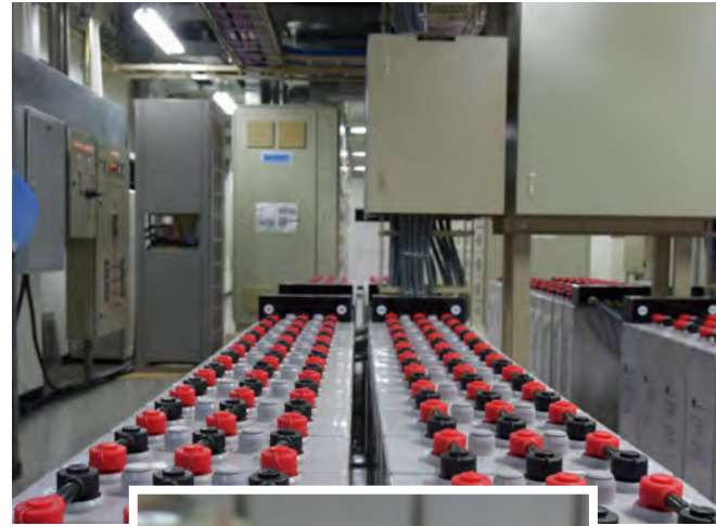
Battery Storage for Cellular Communications Switchboard
