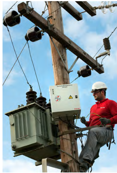
Installation of Voltage Protection
