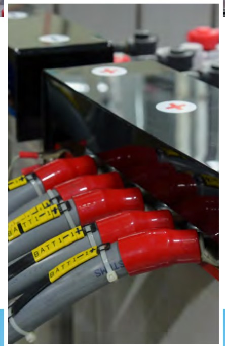
Battery Storage for Cellular Communications Switchboard
