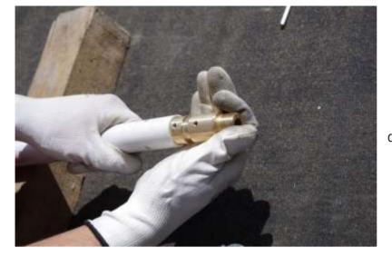
4. Put the brass connector all the way down in to the insulation bar.
