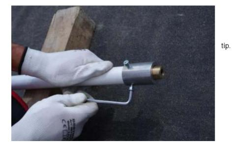
6. Tighten all screws to the insulation bar
