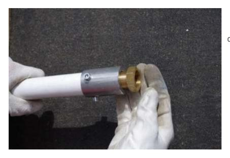
7. Put the brass nut on the brass connector thread and tighten it.
